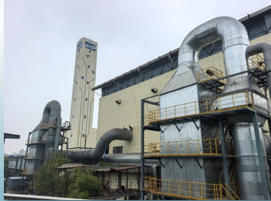
Image: A newly installed flue gas SCR denitrification facility by an enterprise in Zhejiang
